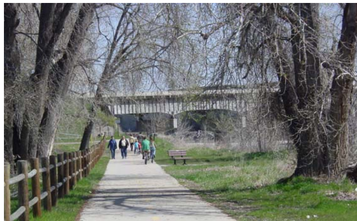
Trail along Yellowstone River through Coulson Park Interstate 90 Bridge in background
