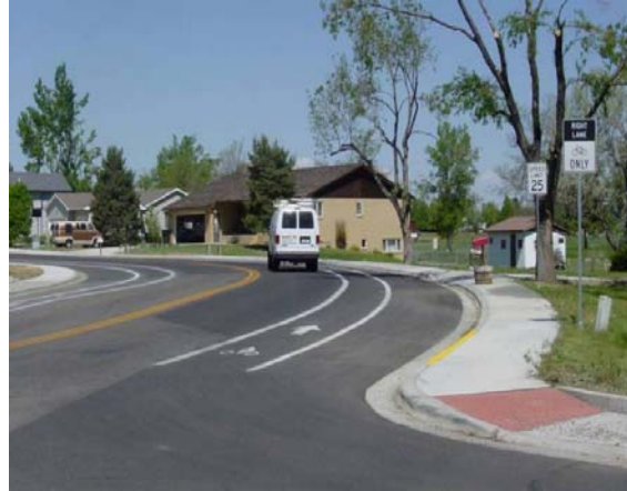
Lake Hills Drive built with bike lanes and parking.
