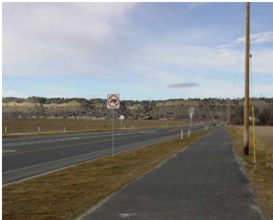
Zimmermann Road built with multi-use trail
